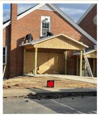
The drains for the basement bathrooms are waiting on inspection before the new concrete can be poured. The new entrance is under roof and the old door gets a new roof to match. The painted open ceiling (below) provides additional brightness to the basement fellowship hall.
